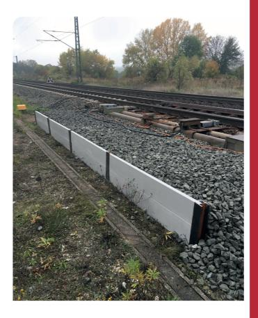
Fire protection classification:K1 (DIN 53438 part 2)Fire behaviour:B-s2,d0 (DIN EN 13501-1)Production control according to DIN 13706Developed according to DBS 918 010 (gratings and<br/>construction profiles made of glass fibre reinforcedplastic in constructive engineering)DB guideline 836.4304 (cycle path constructions)
